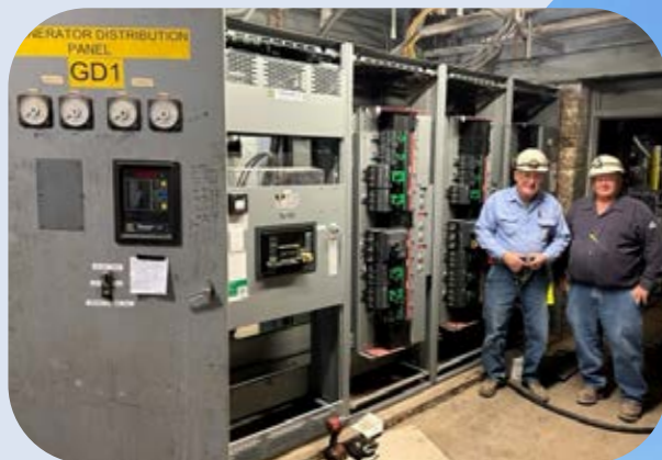
ABOVE Paul Regnerus, left, and Tom Gracias, both Electrical-Instrumentation Technicians at Michigan Sugar Company's Caro facility, stand next to the newly upgraded turbine generator switchgear.
