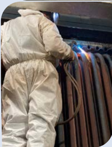
ABOVE A $585,000 boiler retubing project is taking place this inter-campaign on the dual fuel natural gas and oil-fired boiler that has been part of the Caro factory since the 1970s. The boiler produces 150 pounds of steam.
