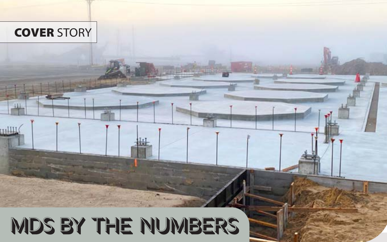
LEFT Foundations and pads for equipment were poured in the fall of 2022 at the MDS project site in Bay City.
