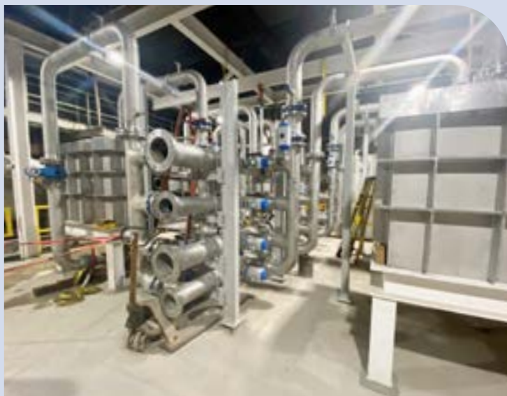
ABOVE A $4 million project to install new juice softening equipment at Michigan Sugar's Caro factory is ongoing. Once operational, the system will improve operations, limit evaporator boil-outs, and generate soft molasses for the desugarization expansion in Bay City.
