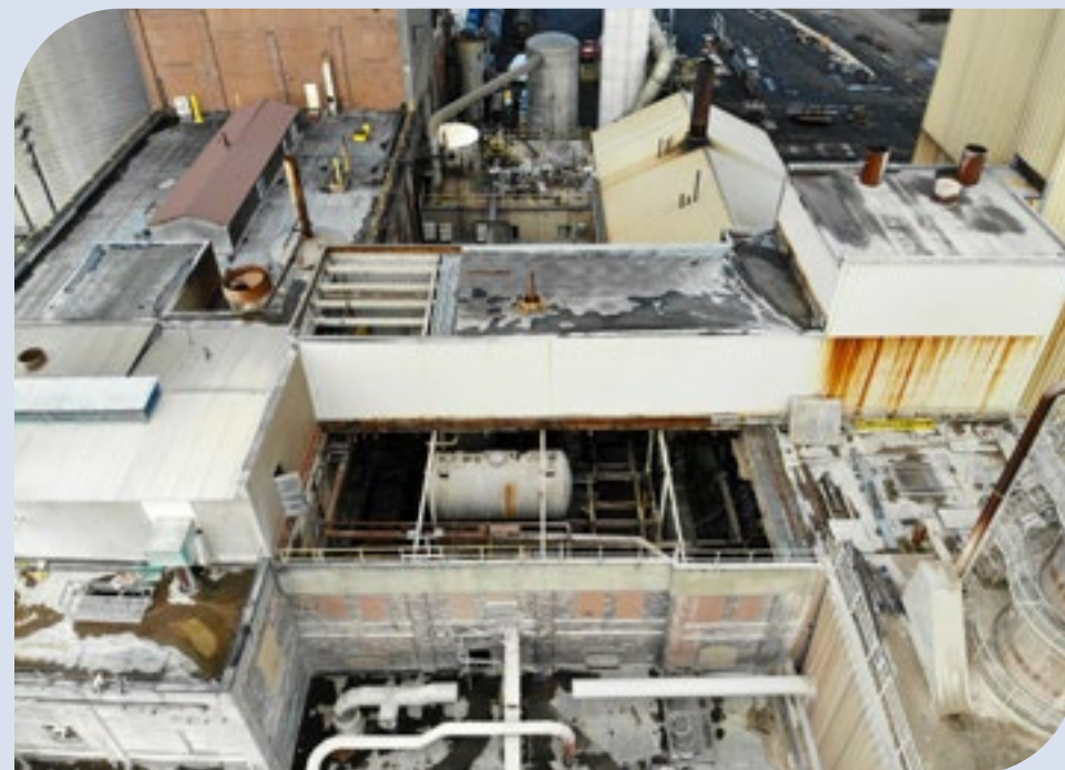
ABOVE Here is a look inside the pulp press building at Michigan Sugar Company's Sebawaing factory. The roof of the building has been removed to allow for installation of several pieces of equipment, including a new pulp press, juice softening storage tanks, and a press water infection control system.
