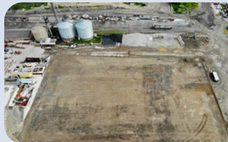
ABOVE This aerial view shows a 114,700-square-foot section of the sugarbeet transfer slab at Michigan Sugar Company's Sebawaing factory where new concrete is being poured this summer. The concrete poured will measure 10 inches in thickness.
