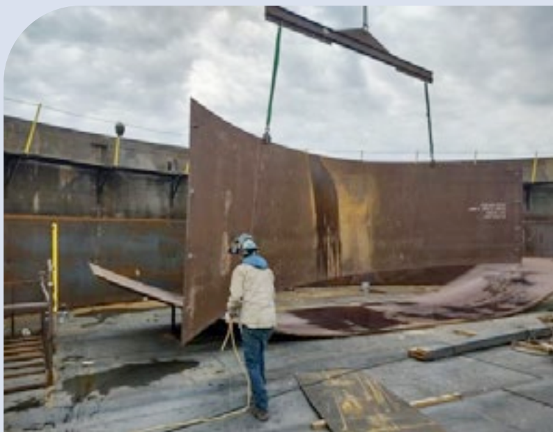
ABOVE Here is a look inside the new 2-million-gallon molasses tank being constructed this summer at Michigan Sugar Company's Croswell facility.
