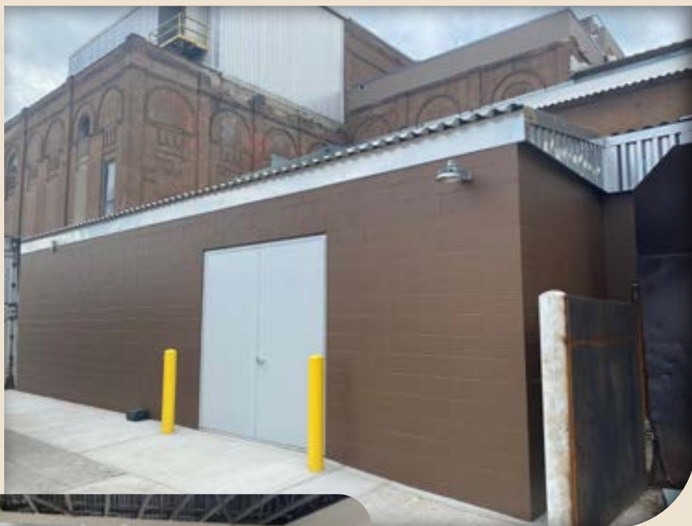
ABOVE/LEFT A new power distribution house at Michigan Sugar Company's factory in Caro includes new switch gear and a transformer. The house provides a clean environment aimed at extending the life of those assets.
