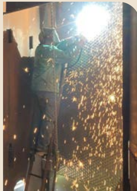
RIGHT A contractor installing one of 38 new heating plates around the inside circumference of the steam dryer.
