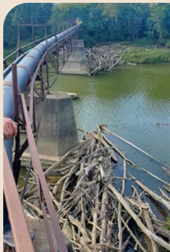
ABOVE/TOP Engineering plans for upgrades to the trestle bridge that spans the Cass River at Michigan Sugar Company's Caro factory. BOTTOM The trestle bridge houses several pipelines connecting the factory to the water treatment ponds. After more than 50 years of service, upgrades are needed to maintain the structural integrity for continued support of the piping.
