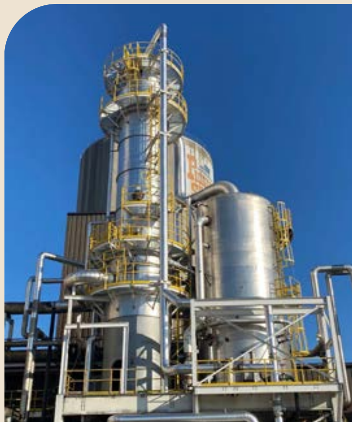
ABOVE A new 40,000-square-foot evaporator and reconfiguration of the evaporator train is designed to maximize throughput and steam efficiency for the factory.
