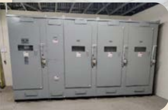
ABOVE/LEFT A new power distribution house at Michigan Sugar Company's factory in Caro includes new switch gear and a transformer. The house provides a clean environment aimed at extending the life of those assets.
