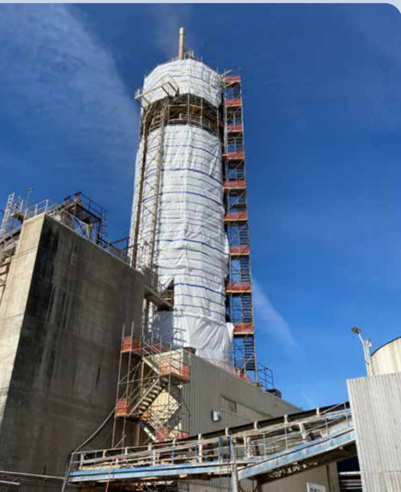
Work to replace significant sections of the steel shell and walkways of the lime kiln began this past summer. The project also involves repainting the lime kiln.
