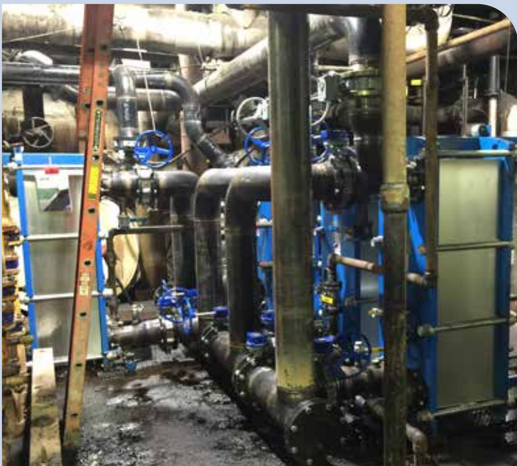
Sebewaing's new thin juice heating station, complete with highly efficient plate and frame exchangers to replace non-serviceable shell and tube exchangers.
