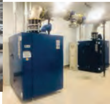
LEFT Major upgrades to the aeration ponds include the addition of two Aerzen turbo blowers spinning at 20,000 RPMs.
