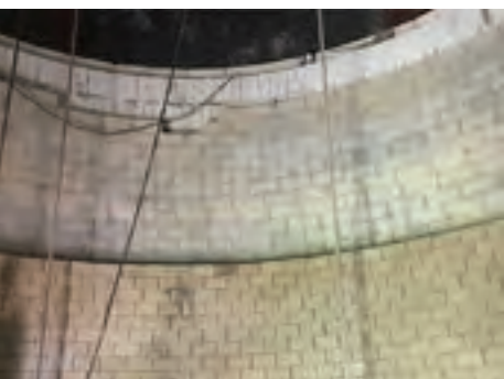
The Eberhardt lime kiln is being relined with new refractory.
