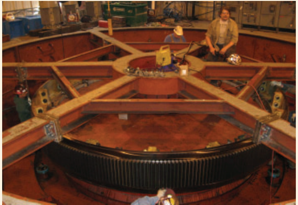
Diffuser bullgear replacement at Sebewaing.
