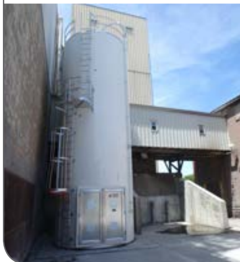
LEFT New bulk soda ash tank.
